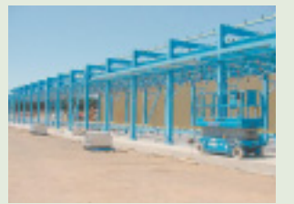
Part of the impressive 40 bay Sling Sorter under construction.
